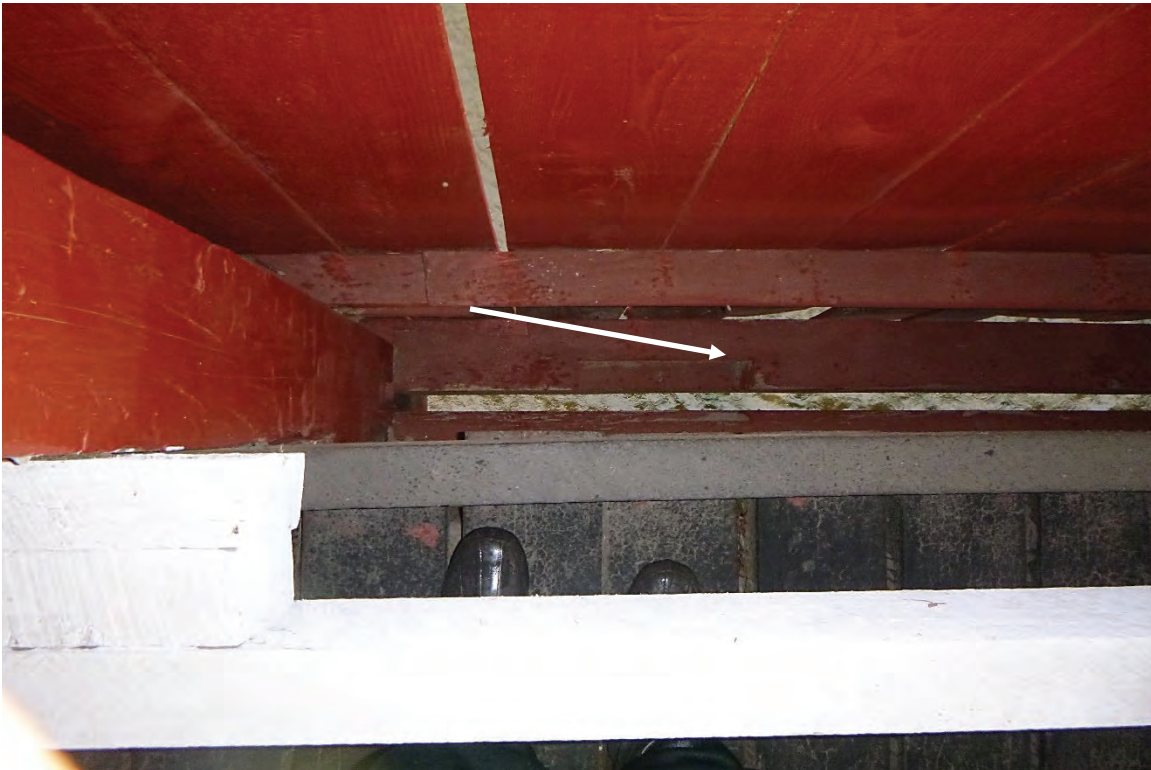
MISSING LOWER LONGITUDINAL KNEE BRACE AT L5 LEFT TRUSS
