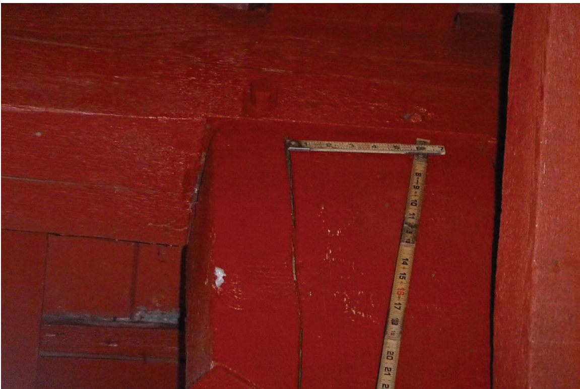
SPLIT IN VERTICAL U5L5 RIGHT ABOVE DIAGONAL NOTCH
