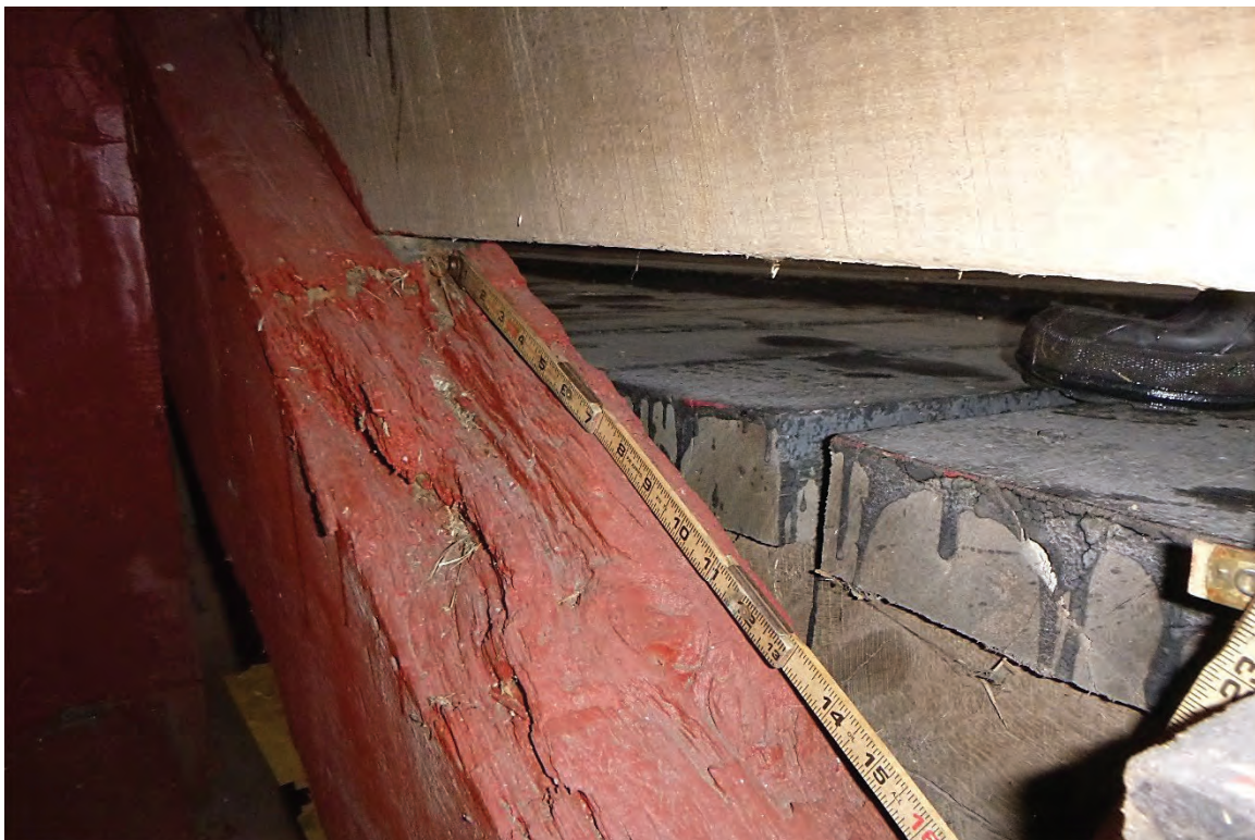
DECAYED INTERIOR ARCH MEMBER AT FAR RIGHT
