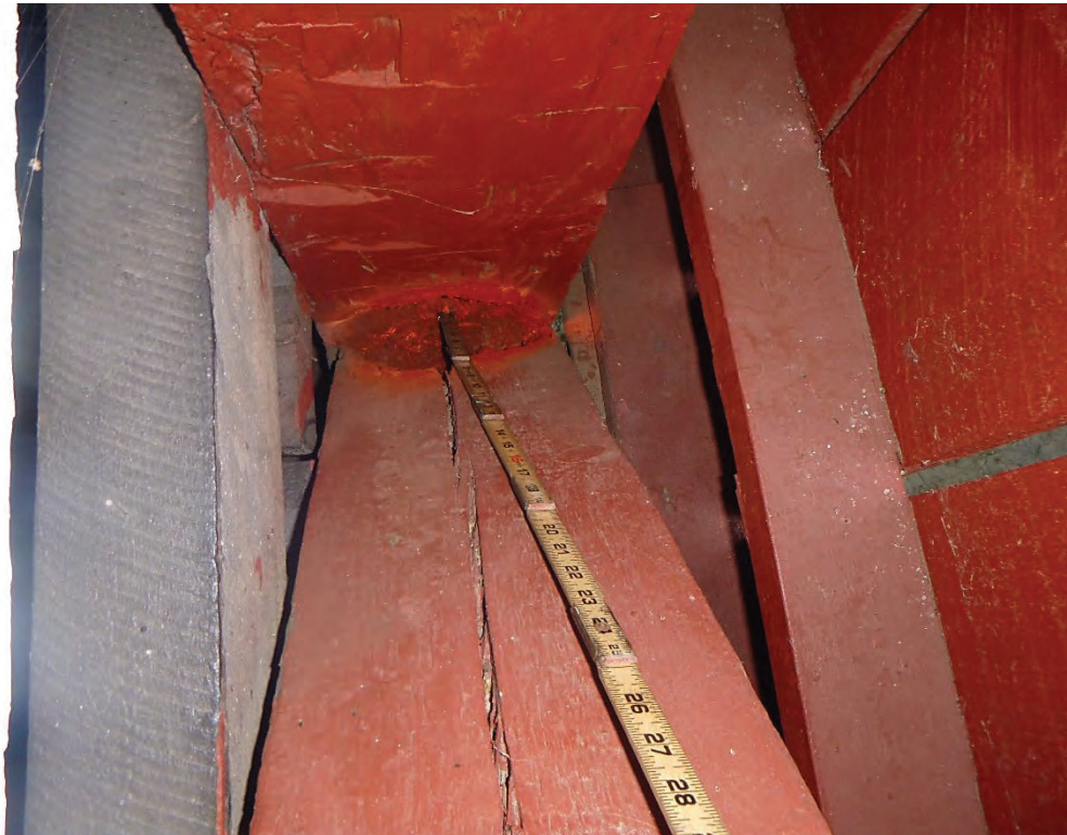
DECAYED VERTICAL AND DIAGONAL MEMBERS AT L6 RIGHT TRUSS
