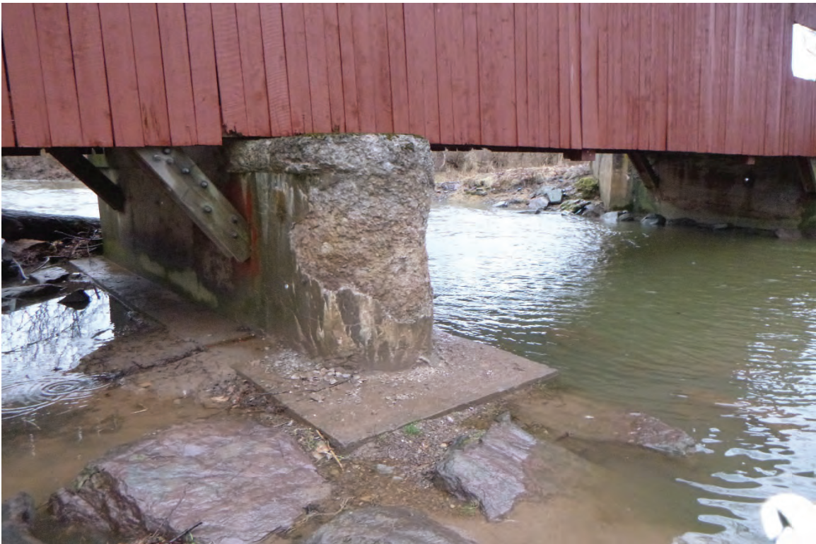
DETERIORATION OF DOWNSTREAM END OF PIER
