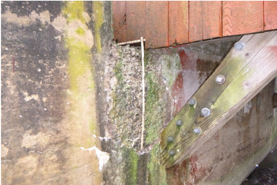
CONCRETE DETERIORATION AT THE FAR ABUTMENT
