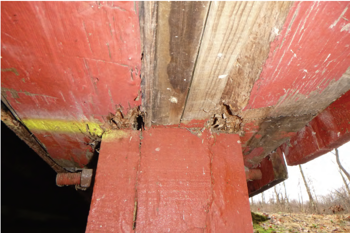
DECAY IN THE EXTERIOR LOW CHORD AT FAR SIDE OF U1L1 Left
