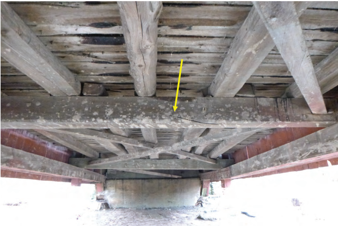
HEAVY CHECK ON FAR SIDE OF FLOORBEAM 2
