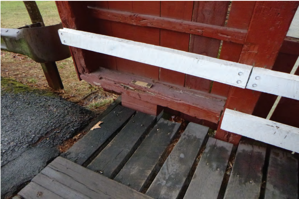
DECAY IN SILL PLATE AT FAR RIGHT PORTAL
