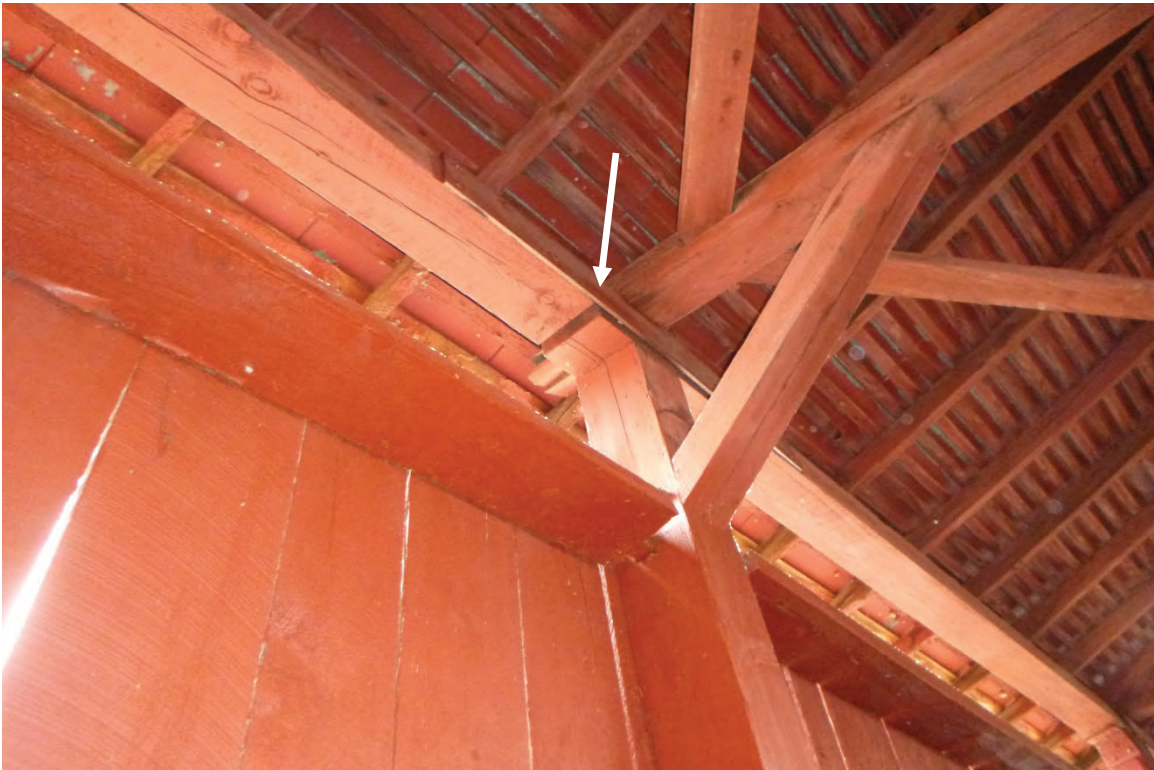
MISALIGNED HEADER BOARD AT U4 LEFT
