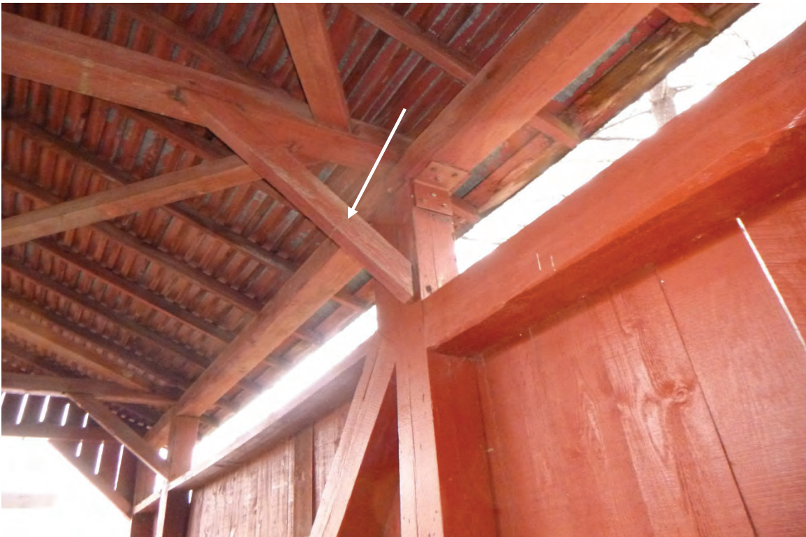
LOOSE KNEE BRACE AT U5 RIGHT
