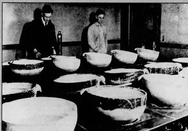
Many scientists and workers at Standard Chemical died from cancers and anemia caused by exposure to radium, which took several steps to produce, such as fractional crystallization, above.
